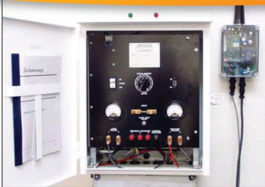
When using an impressed current cathodic protection system to protect a steel UST system from corrosion, it must be active constantly — 24 hours per day, 7 days per week, every day of the year. In addition, the
