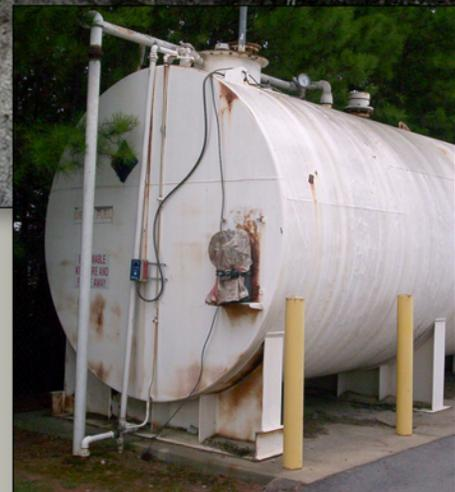
spill container does not contain water or product. The inspector also verifies that no debris or fire hazards exist in the containment area, that tank attachments are secure and free of corrosion, that a liquid level gauge is functioning properly, and more.
